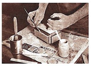
Above: Edges of pieces are touched up with paint before inserting the mitered "in between" sections.
