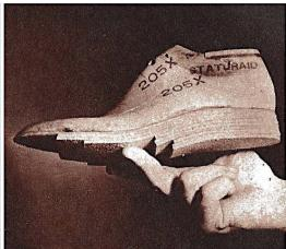
Slanting inner soles of cork are used to make "high heels" inside men's shoes. Below, a cobbler and 26 cork soles for one shoe.
